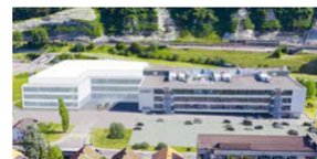
Building permit granted to expand production capacity in Flamatt
